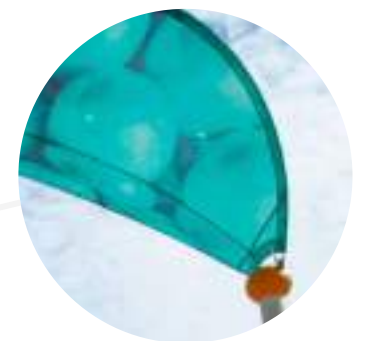
Roof Printable on both sides, dirt-repellent, recyclable and UV light resistant mesh fabric in the leaf like roof construction
